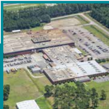
CONWAY, SC Steel Foundry and Manufacturing Plant
