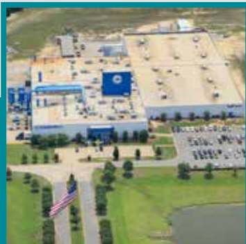
PAGELAND, SC Bronze Foundry and Manufacturing Plant
